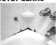
obvious we can see that is causing the leaking and damage to the ceiling below. After opening ceilings, etc., the cause of the leak turns out to be a bathtub that is not properly caulked allowing water to seep below. Caulking turns brittle and cracks and no longer serves as a seal, opening the way for mildew to take hold or for water to seep through and turn wallboard and framing mushy.
